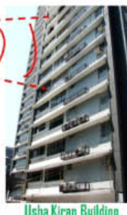
Usha Kiran Building
